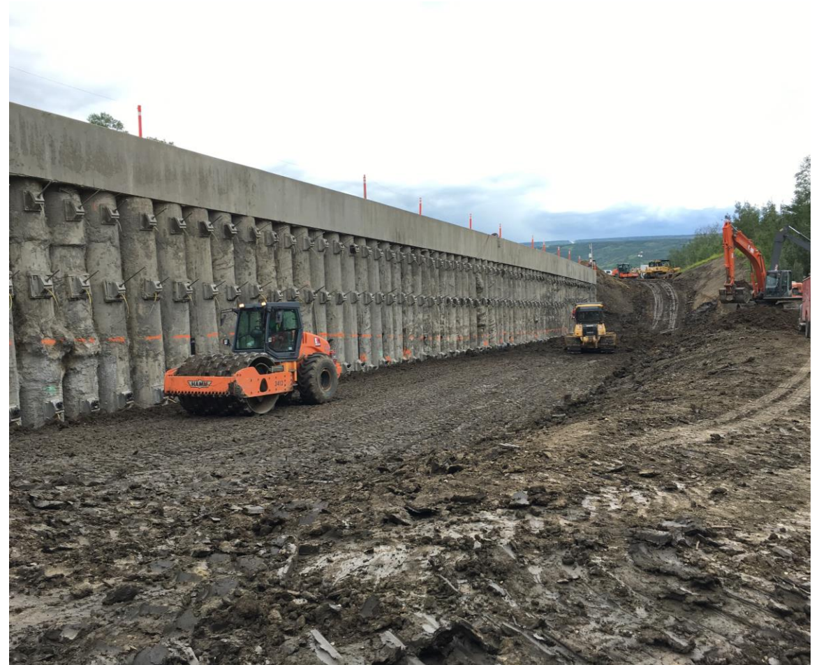
Construction Inspection at a CIP Secant Pile Wall in Peace River
